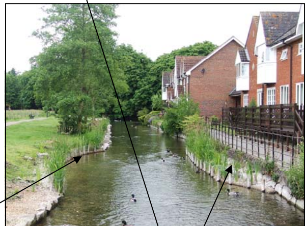
New berm constructed from 'as dug ballast with coir roll and additional planting. Photo taken in June 2009
